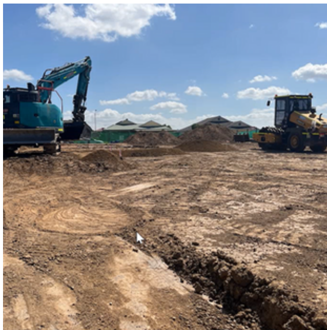
Singleton Refuge starts construction
